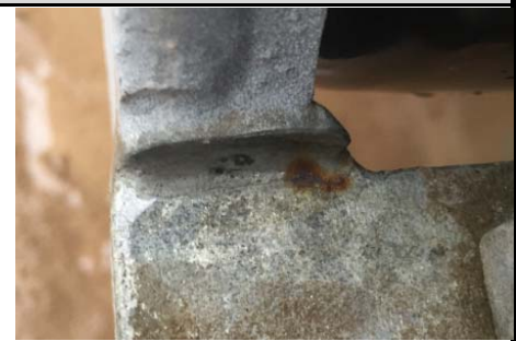
Crack Developing in Caster
