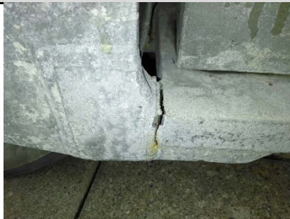
Large Crack in Caster
